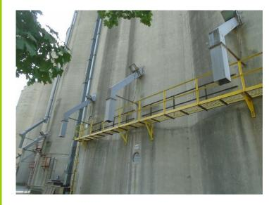
Yes, this **Safety Made Simple** partner recently installed a catwalk with guardrail and self-closing safety gates to access their loadout spouts. Prior to installation, employees used extension ladders to access platforms located at each spout.
